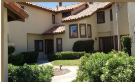
Greens units with window accents
